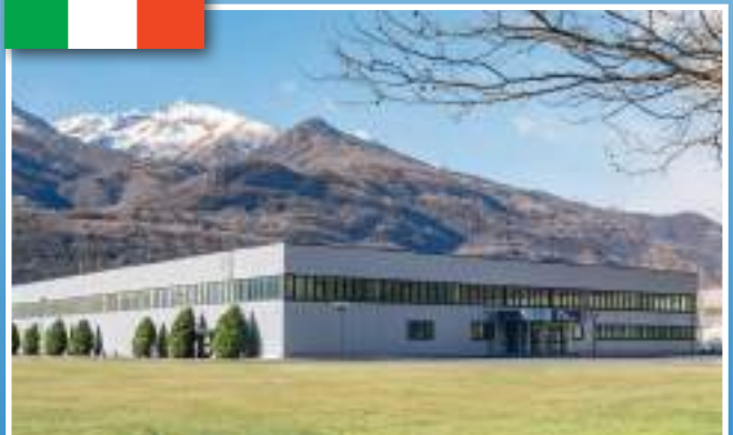
AUTOBLOK manufacturing plant Caprie-Torino
